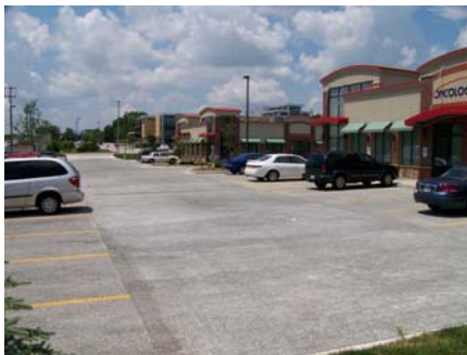
Enhanced Porous Concrete Paving
