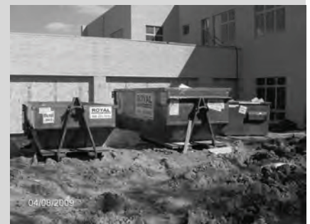
Construction waste recycling at Holy Wisdom Monastery
